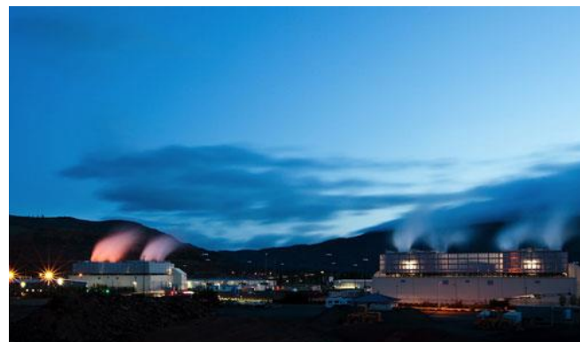
Water vapor rises above the cooling towers in The Dalles data center in Oregon. These plumes of water vapor create quite a mist at dusk.
